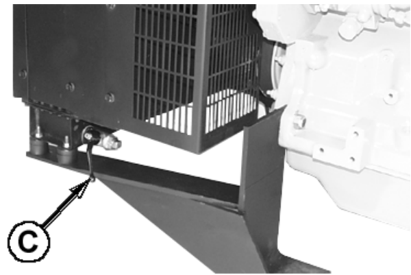
Radiator Drain Valve
